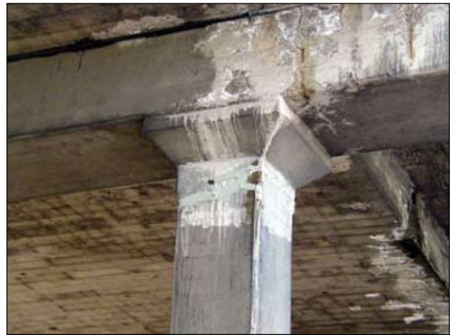
The South Park Bridge in Seattle suffered extensive damage. Above is one of 22 columns that cracked in the earthquake. Epoxy was injected to shore up the structure. Crews worked round the clock to repair this and other structures throughout the area. Photo: King County
