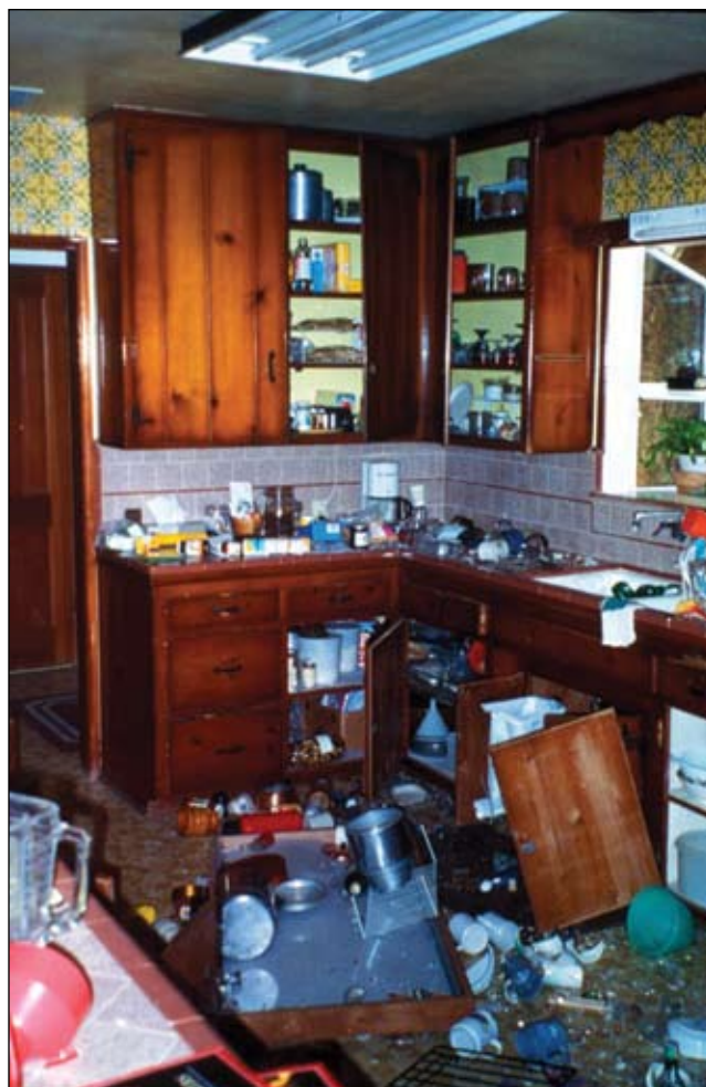
Falling walls are not necessary for injuries to occur. Kitchens can be a place of major nonstructural damage. Glassware, dishes, and food containers can fall from shelves. Cleaning supplies can fall off shelves and break. Mixing of some chemicals, like chlorine bleach and ammonia, can produce serious hazards. Photo: P. W. Weigand, California State University at Northridge
